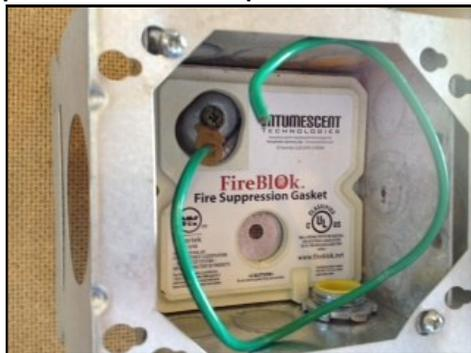
FireBlok® Gaskets are designed to fit easily into electrical boxes. The pre-molded openings insure metal to metal contact while assuring wiring is accessible at all times per NEC.
